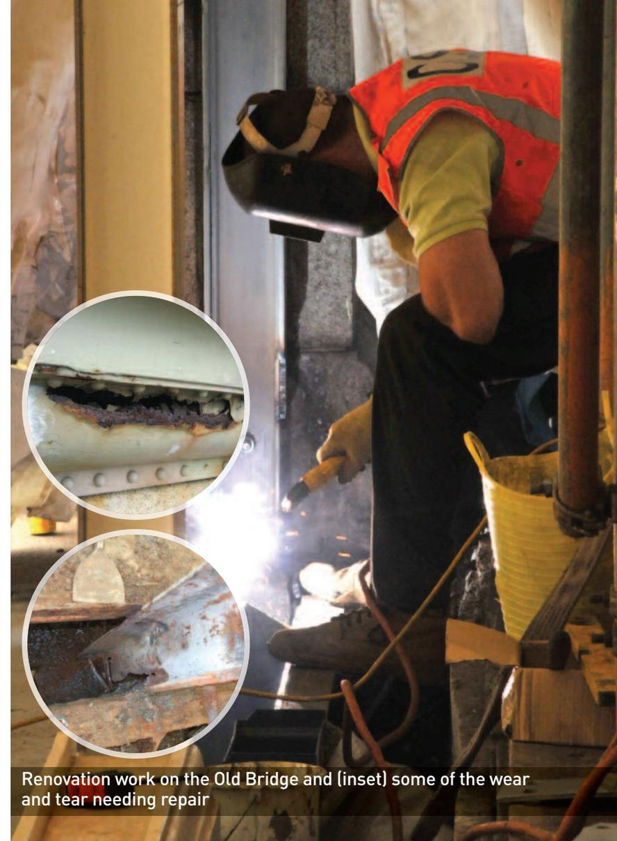
Renovation work on the Old Bridge and (inset) some of the wear and tear needing repair
